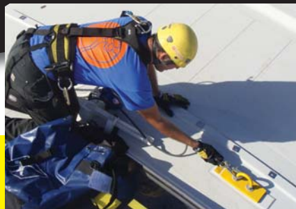
Anchor rescue carabiner to the nacelle anchor point .
